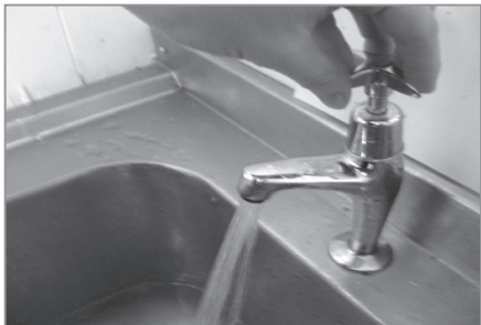
Fill sinks with clean water and empty to flush through unit. This keeps freshwater in tank. Always ensure water level is reaching wheels.
